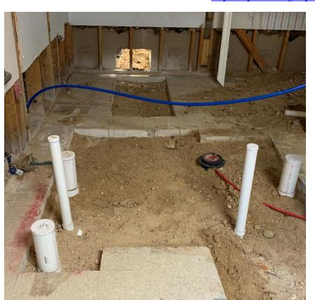
Big progress this past week. The pipes in the trenches were approved by the city inspector. The pipes were covered with existing dirt preparing the way to lay down the rebar, which supports the concrete flooring
