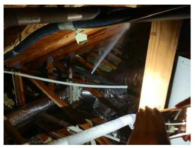
split and ran unabated for the better part of 2 days during the coldest part of the storms. City Wide of Austin came the next day to remove much of the debris that had showered down from the ceiling carried by the water and started drying fans.
